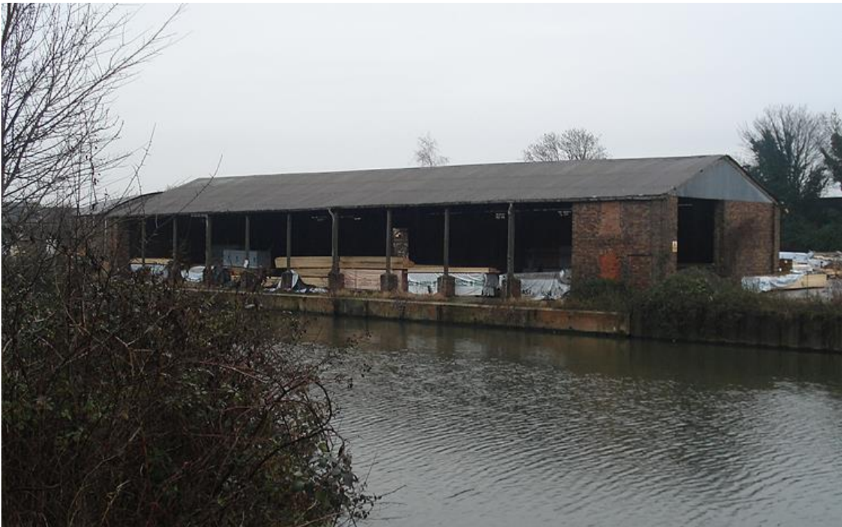
Plate 5 The northern salt warehouse on Bristol Road, from the south west
