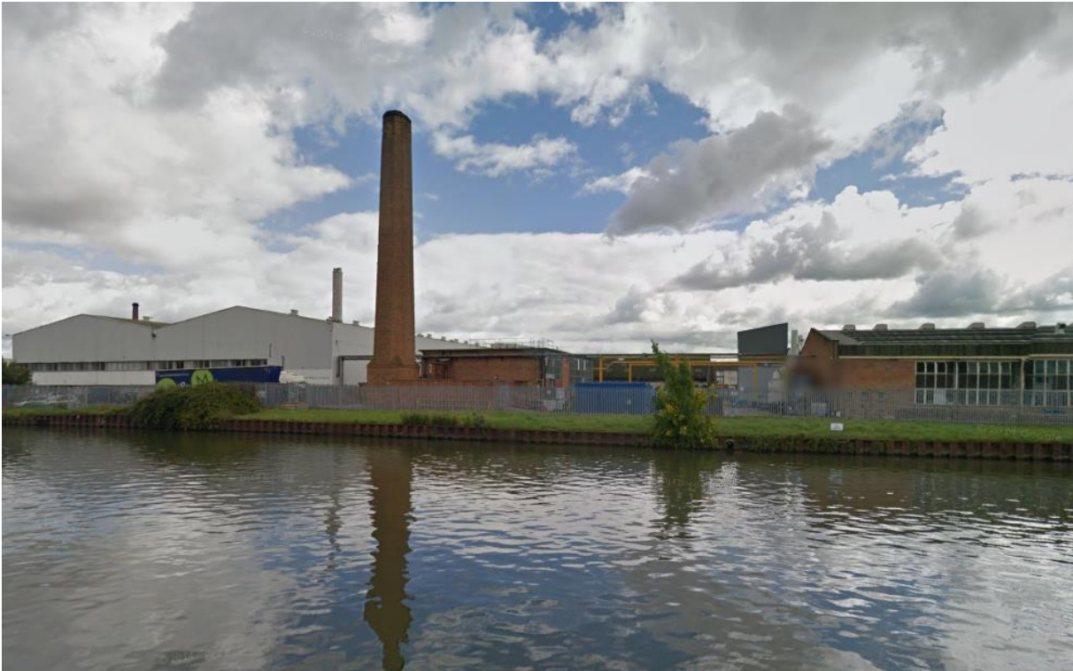
Plate 10 Mill Place Chimney from the west
