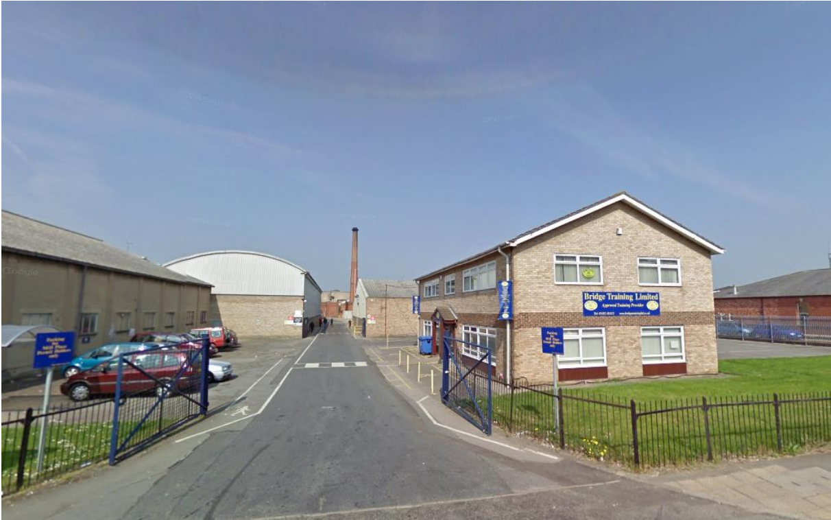
Plate 7 Madleaze Chimney from the east before the height was lowered.
